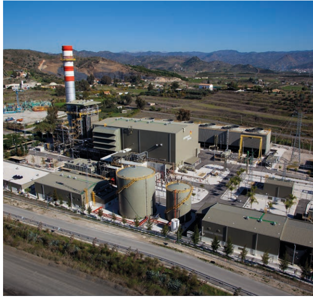
Combined cycle power plant in Malaga, operated by Naturgy
